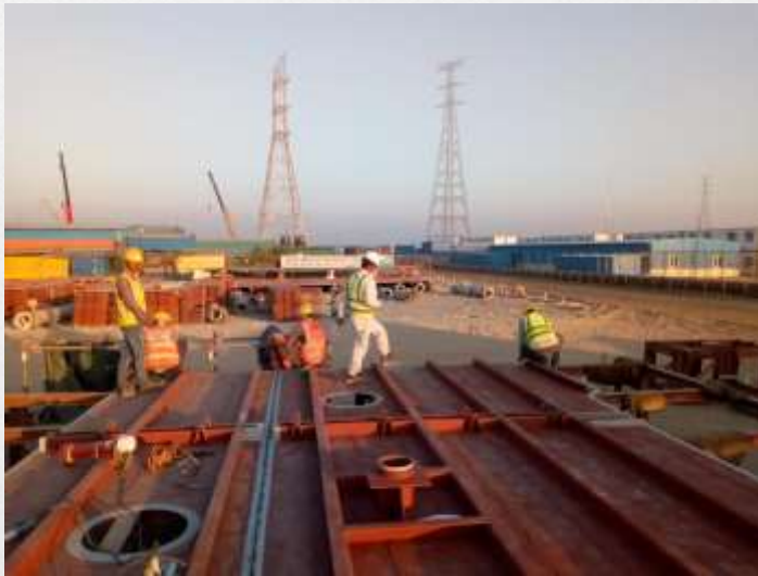
ECO CASING PLATE PRE ASSEMBLY
