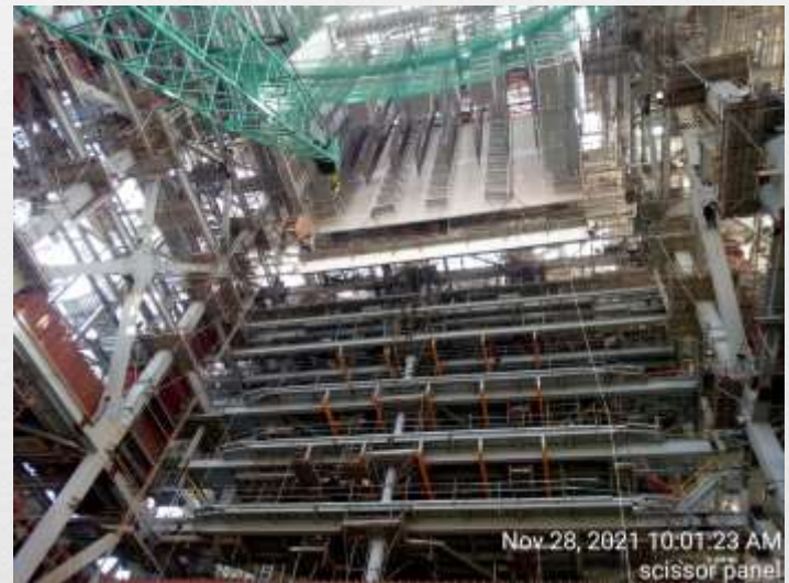
FURNACE FRONT SCISSOR PANEL (INTERMEDIATE HEADER) LIFTING
