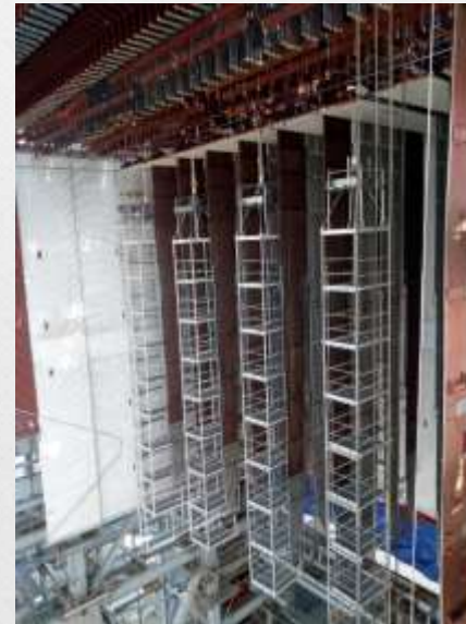
FURNACE ROOF PANEL LIFTING WITH HANGING SCAFFOLDING
