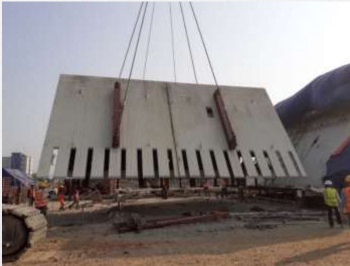
NOSE PANEL SHIFTING FROM PRE ASSEMBLY AREA TO BOILER CAVITY AREA
