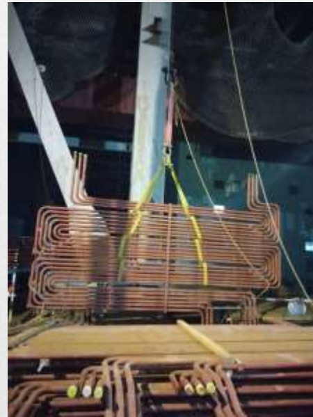
PRIMARY REHEATER COIL LIFTING
