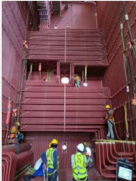
PRIMARY SUPERHEATER COIL LIFTING
