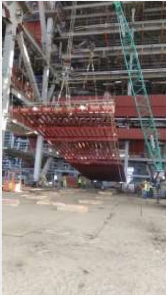
HRA FRONT WALL PANEL LIFTING
