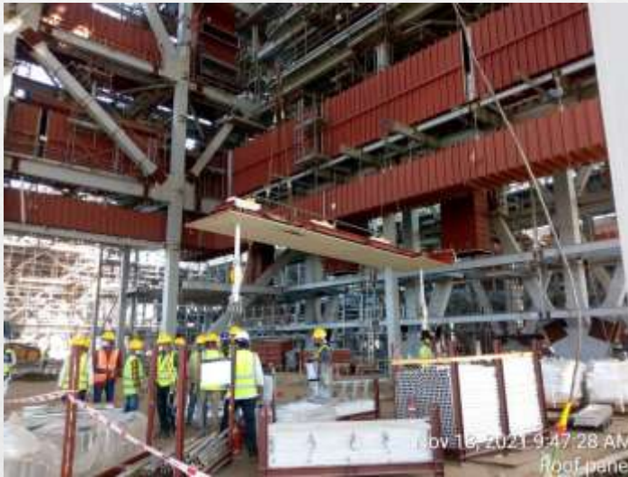
FURNACE ROOF PANEL GROUND ASSEMBLY WITH HANGING SCAFFOLDING
