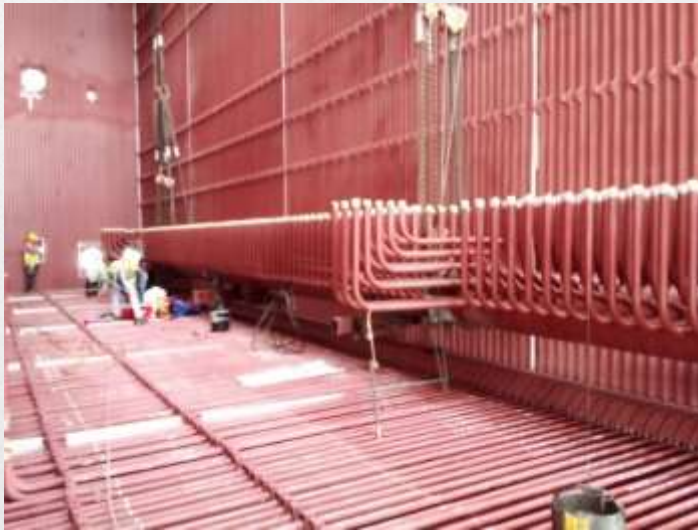
PRIMARY SUPERHEATER INLET HEADER ALIGNMENT
