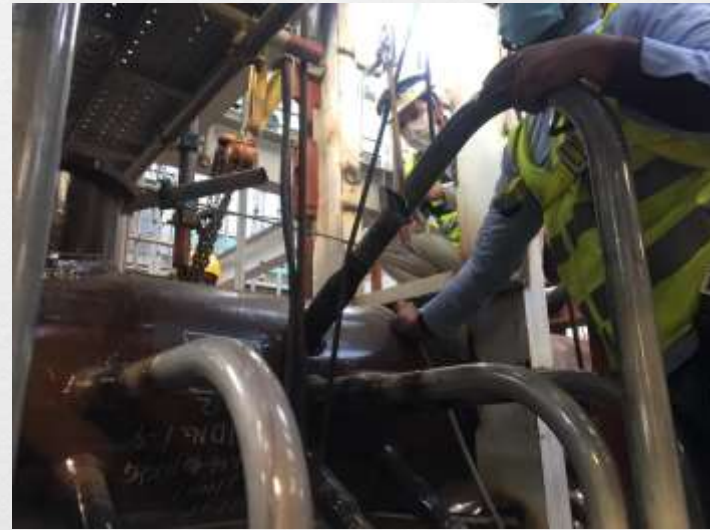
FINAL SUPERHEATER COIL HEADER ALIGNMENT DONE
